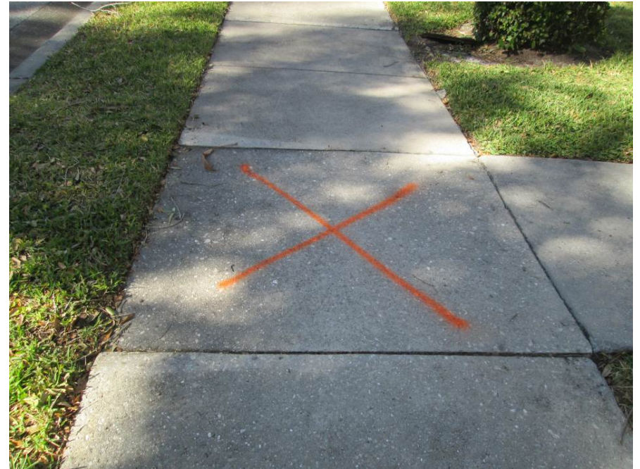
Replace 5' x 5' panel in front of lot 57 Whitehead St
