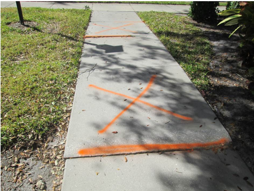
Replace 2 ea 5' x 5' panels lot 94 Whitehead St
