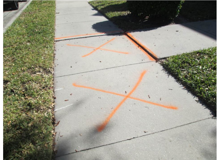
Replace 10' x 5' panel in front of lot 97 Whitehead St
