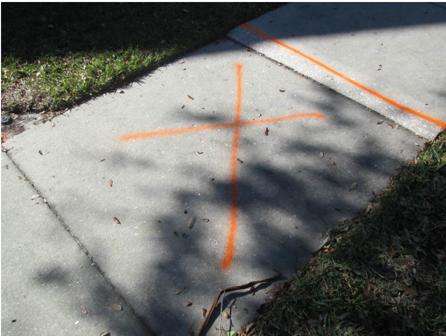
Replace 6' x 5' panel in front of lot 96 Whitehead St
