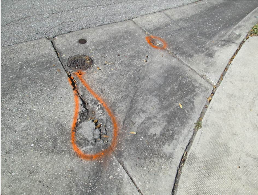
Chip loose concrete, epoxy grout NE corner Whitehead & Hemmingway
